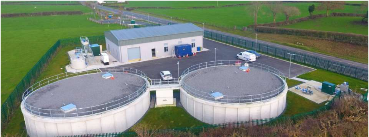
Figure 4: Completed Water Treatment Plant at Gowran, Co. Kilkenny.
