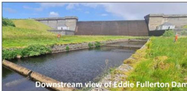
Figure 2: Eddie Fullerton dam completed in 1997 to supply Buncrana Co. Donegal
